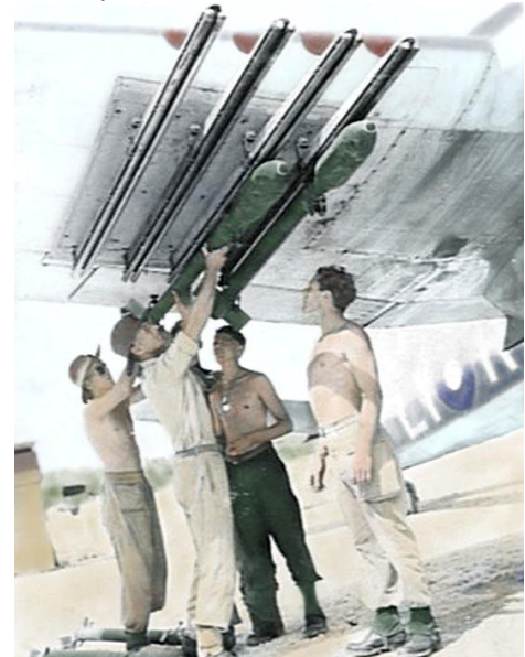
A19-192 EH-T Mk.X of 31SQN at Coomalie NOV 1944 with the introduction of the 3-inch / 60-pound rocket From left: navigator F/O S Greene, LAC Forest, and Greene's pilot F/O A Cobb
