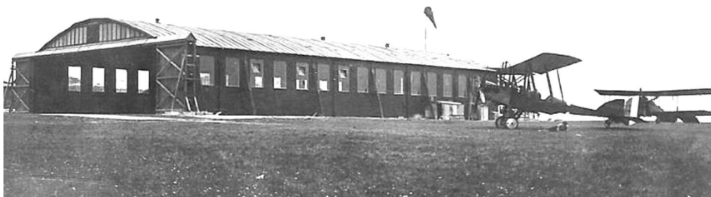
Six of these hangars were constructed at Harlaxton from OCT 1916 – the same design as Yatesbury airfield, above
